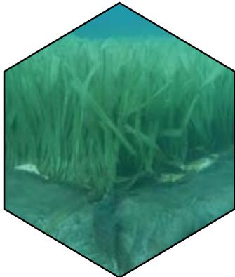
Artificial seagrass used to prevent scour (sediment erosion) around sub sea installations (pipelines, cables).
